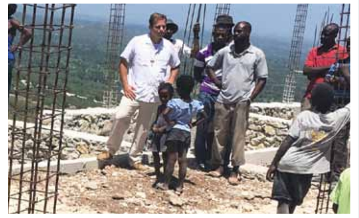
Fr. Michael Mitchell, LC, with Haiti villagers, on the foundation of their new school.
