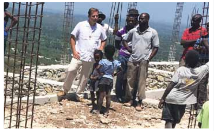
Fr. Michael Mitchell, LC, with Haiti villagers, on the foundation of their new school.
